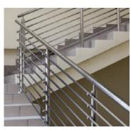
ets, and fittings that can be used to assemble — without welding — almost any type of interior or exterior handrail. Tubing options include three diameters, two wall thicknesses, and two finishes. Prices range from \$6 to \$19 per lineal foot.
