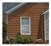
NichiFrontier Siding has the same footprint (91/4 inches by 8 feet) and cedarlike appearance as the company's 1/2-inch-thick Sierra Premium boards but is only 7/16 inch deep. It can be ordered with a factory-prime coat or finished in one of four stain colors. Contractor pricing runs about \$3 per square foot.
