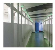
Tooshlights is a public restroom lighting system that communicates stall occupancy. The LED lighting system expedites wait times, enhances security, and assures privacy. Wireless technology triggers the light to change to red or green and can be used for both regular and handicapped bathroom stalls. TOOSHLIGHTS by TOOSHLIGHTS. Circle 201. www.tooshlights.com
