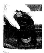
Step 8. Reinstall the Flush Valve Cartridge (FVC) Assembly. First, insert the cartridge into vessel and, while gently pushing down on the cartridge turn the cartridge clockwise \_ turn to lock the FVC into position with connector ports aligned and facing forward, indicating that the locking are now aligned. Turn on the water check carefully for leaks.
