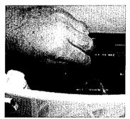
Step c. Disconnect the Dual Flush Control valve orange and blue lines, but rotating the locking tabs downward and pull gently on the lines.
