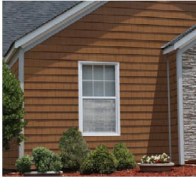
*NichiFrontier Siding* has the same footprint (9 $\frac{1}{4}$  inches by 8 feet) and cedarlike appearance as the company's  $\frac{1}{2}$ -inch-thick Sierra Premium boards but is only  $\frac{7}{16}$  inch deep. It can be ordered with a factory-prime coat or finished in one of four stain colors. Contractor pricing runs about \$3 per square foot.
